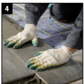
Install floor finish Cover the heating cables with self-levelling compound, sand and cement screed or
