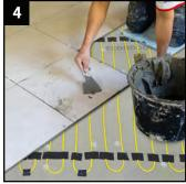
Install floor finish Take images of the installed cables before installing the into position go back and add floor finish. Cover the heating cables with a flexible cement based self-levelling or tile directly on top using a full bed of tile adhesive.
