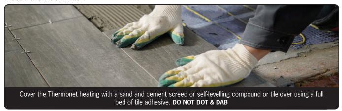
The entire floor heating cable (including the entire cold tail connection and the end termination) needs to be encased in a flexible, cement based compound (No specific brand required). Thermonet can be tiled over directly (ensuring there is a full bed of tile adhesive) or covered in a self-levelling compound or sand and cement screed. For screeds over 20mm thick use the Thermonet 200W/m<sup>2</sup> for optimum performance.
