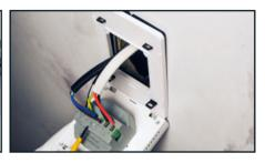
**12. Connect to the power supply** Connect the Thermorad panel lead into the incoming power supply or timer. This work must be undertaken by a qualified electrician and it is important to ensure any electrical connections are accessible.
