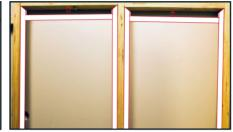
**5. Dual setup for multiple or wide rails** When installing multiple rails side by side or rails over 650mm wide, we recommend the use of two Thermorad panels to increase the heating area. Having a stud running between the two Thermorad's provides an anchor point for the wall sheeting to be fixed to.
